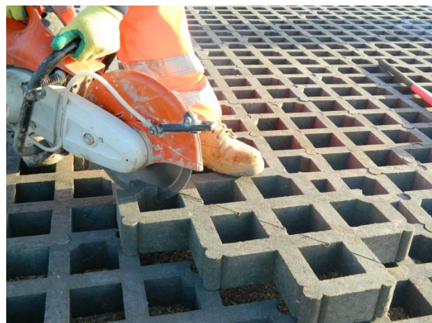
Cutting Truckcell to size
