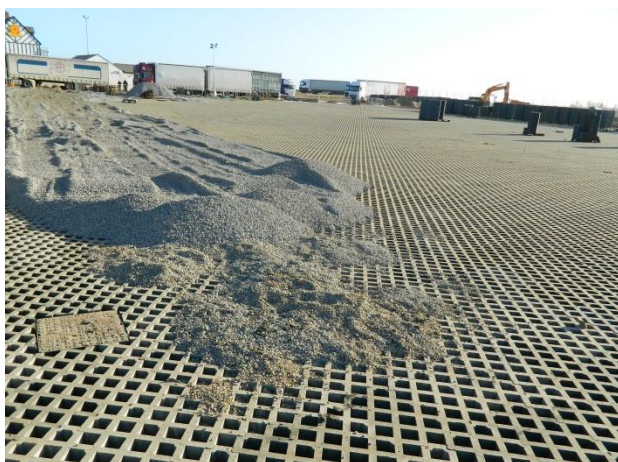
Truckcell being filled with porous angular aggregate.
