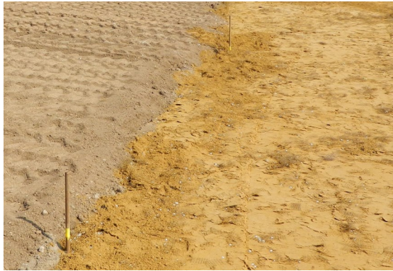
Fig. 5: Maintain accurate levels
