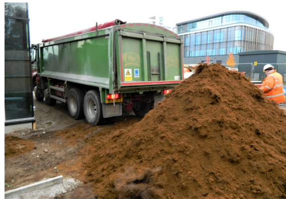
Fig. 2: Rootzone bulk delivery
