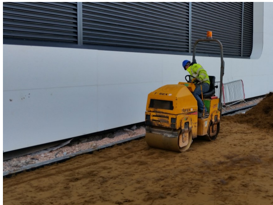
Fig. 6: Rootzone compaction with roller
