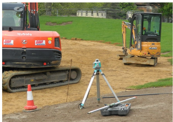
Fig. 3: Set accurate rootzone levels
