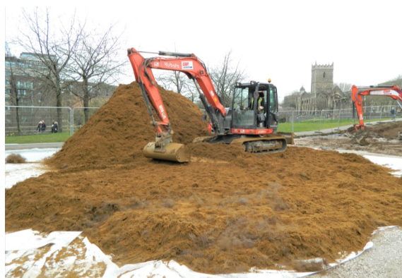
Fig. 4: Rootzone spreading over Terrex NW9
