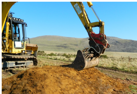
Fig. 7: Rootzone compaction on slopes
