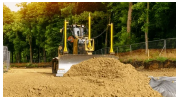
Fig. 8: Dozer spreading aggregate
