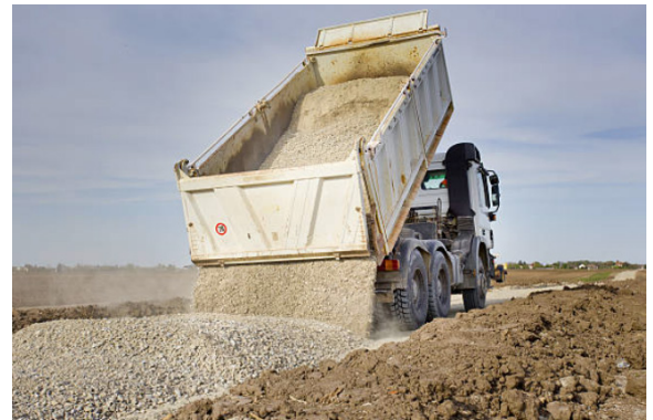
Fig. 7: Dumping of aggregate fill on geogrid
