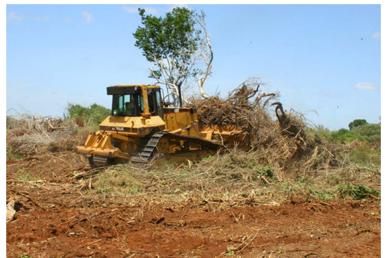
Fig. 3b: Subgrade preparation
