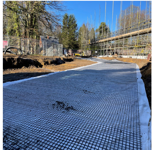
Fig. 5: Application of ABG non-woven geotextile with Abgrid geogrid
