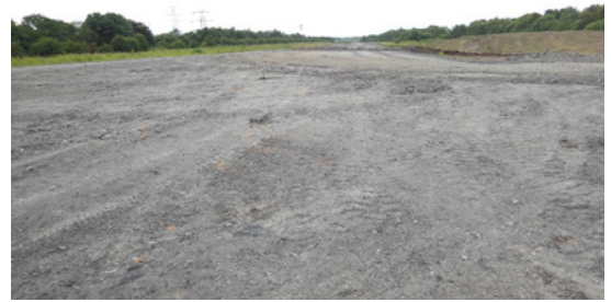
Fig. 3a: Subgrade preparation
