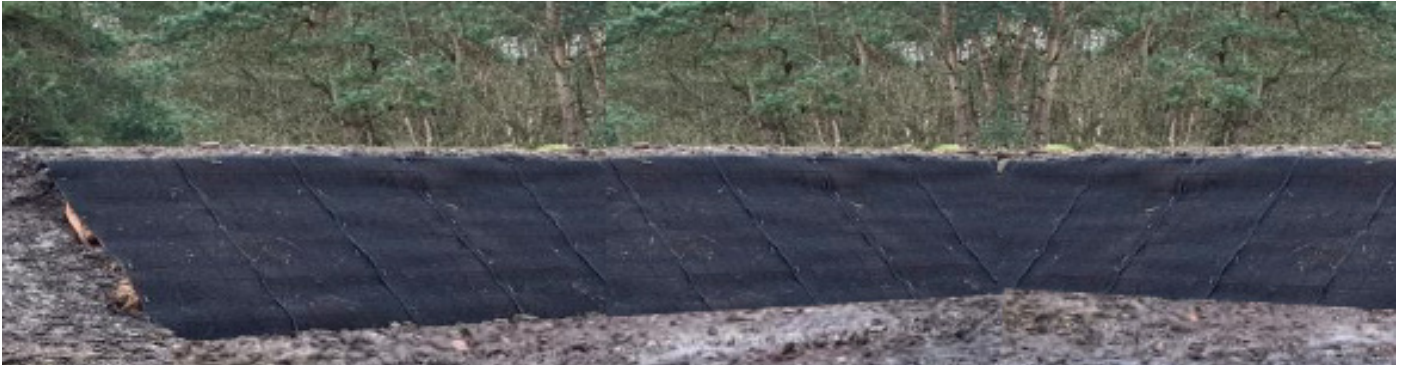
Fig. 9: Completed slope awaiting to be seeded / greened
