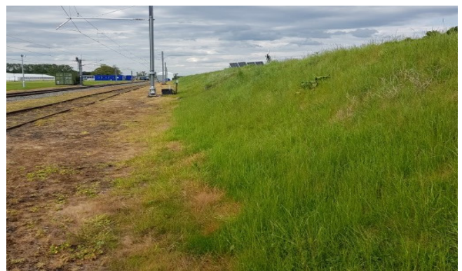
Fig. 2: A completed vegetated slope
