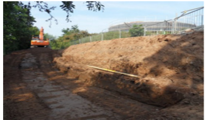
Fig. 1: Cut & prepare site to formation level
