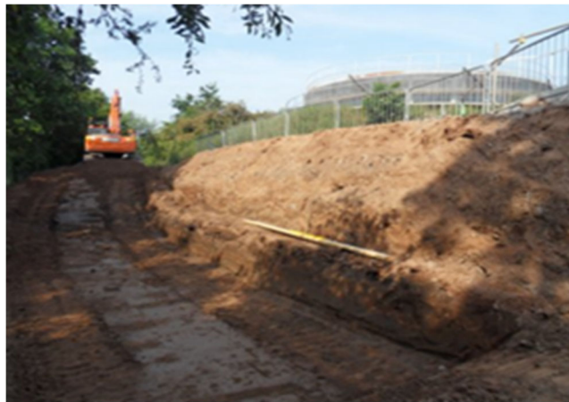
Fig. 1: Cut & prepare site to formation level
