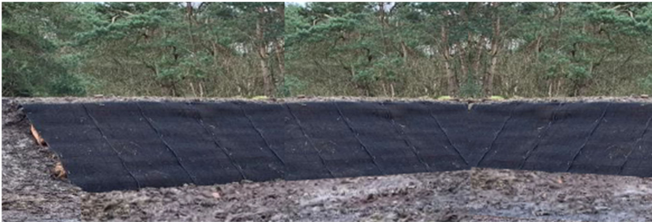
Fig. 9: Completed slope awaiting to be seeded / greened
