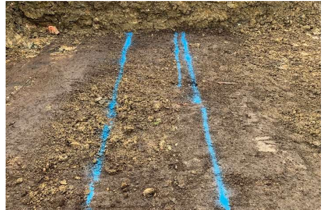
Fig. 4: Cut site to shape with level base in preparation for reinforced slope construction
