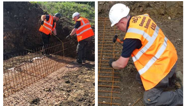
Fig. 4: Cut site to shape with level base in preparation for reinforced slope construction
