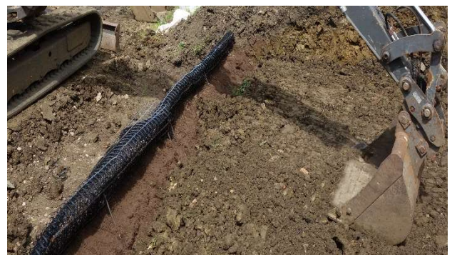
Fig. 13: Brace bars fixed, geogrids tensioned at the back of the slope against layer of fill load to remove slack
