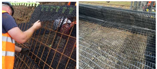
Fig. 10a: Place and fix the vegetation liner at the inner side of the facing mesh using cable ties
