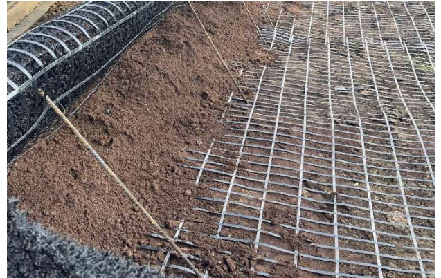
Fig. 12: Topsoil placed and brace bars fixed
