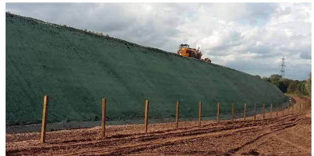
Fig. 17: Slope face after hydroseeding
