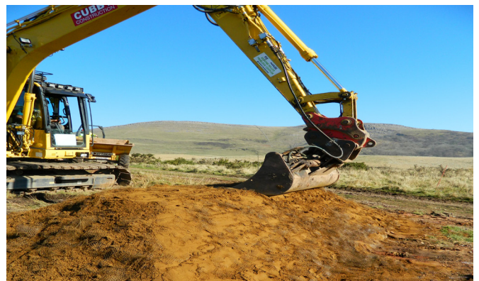
Fig. 7: Rootzone compaction on slopes
