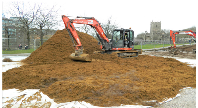
Fig. 4: Rootzone spreading over Terrex NW9
