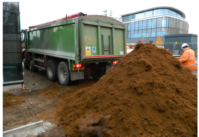
Fig. 2: Rootzone bulk delivery
