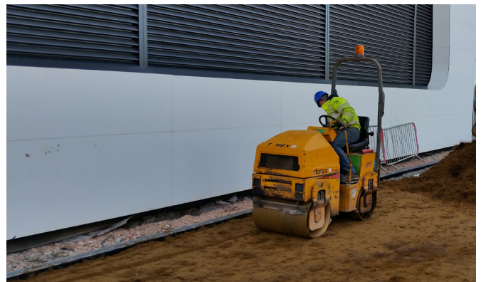
Fig. 6: Rootzone compaction with roller
