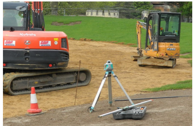
Fig. 3: Set accurate rootzone levels
