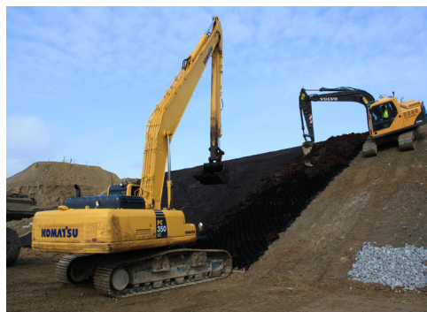
Installation and filling of Erosaweb GWX on 1:2.5 slopes
