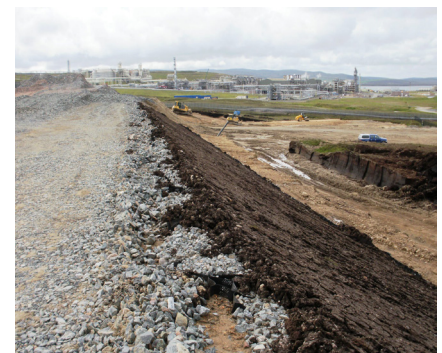
Peat filled Erosaweb provide natural finish on steep slopes
