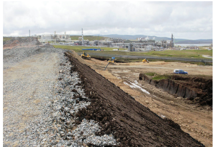
Peat filled Erosaweb to provide a natural finish on steep slopes
