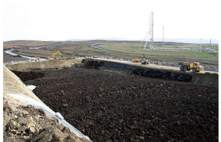
Peat store lined with Pozidrain being filled
