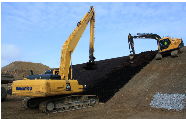
Installation and filling of Erosaweb GWX on 1:2.5 slopes
