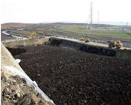
Peat store lined with Pozidrain being filled
