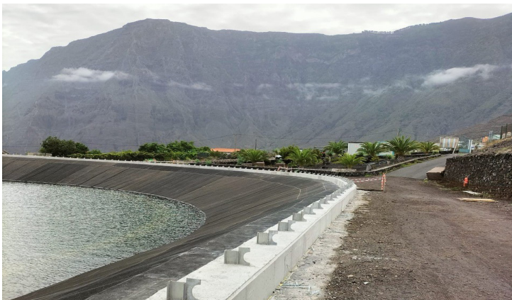
Completed basin lining prior to fabric cover installation
