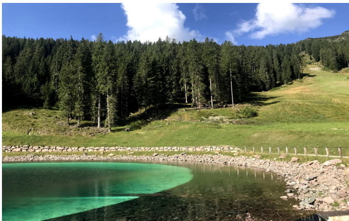
Dual layer of Pozidrain 4SK250/NW8 installed back-to-back to provide groundwater drainage & leak detection functions
