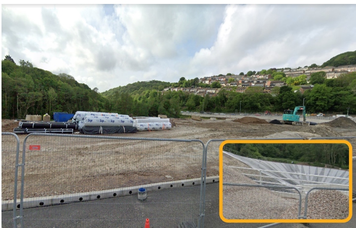
Pozidrain and Trigrid rolls on site & during installation (inset)
