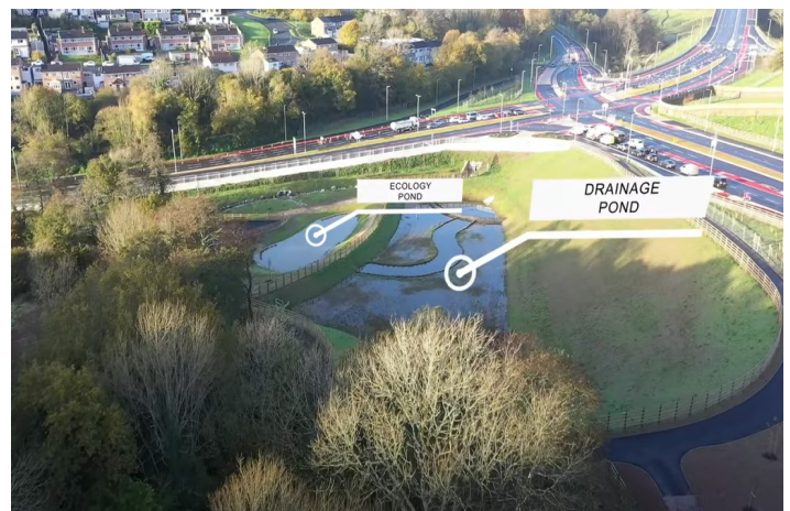
The completed detention ponds at the Forder Valley link road
