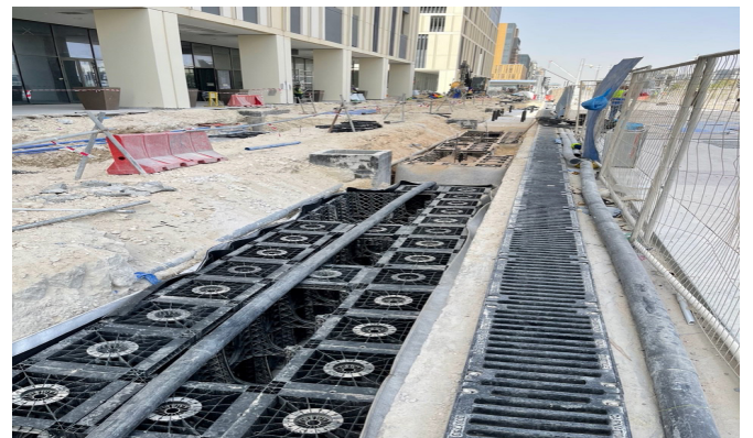
Salt Break barrier lines the soil containment modules as part of the sub-surface irrigation system
