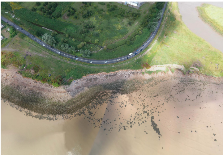
Coastline prior to revetment construction
