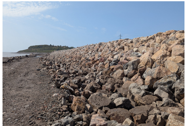
The new rock armour structure installed onto the Terrex CG layer
