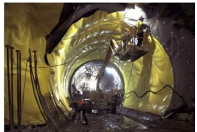
Fig. 6: Cavidrain Liner installed on tunnel walls
