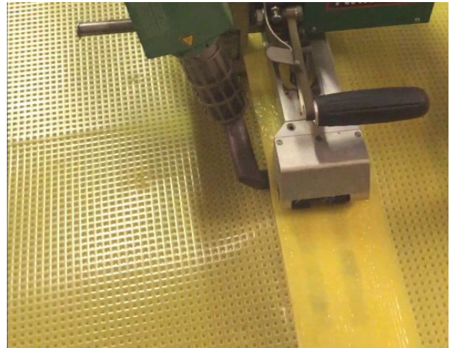
Fig. 7: Double weld on selvedges of two panels
