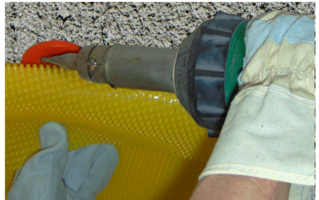
Fig. 5: Cavidrain Liner welding to rondel
