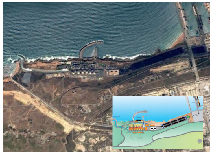
Finished facility with no leachate entering the environment
