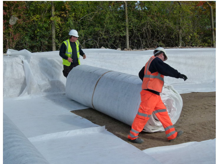
Fildrain Geocomposite drain installation.
