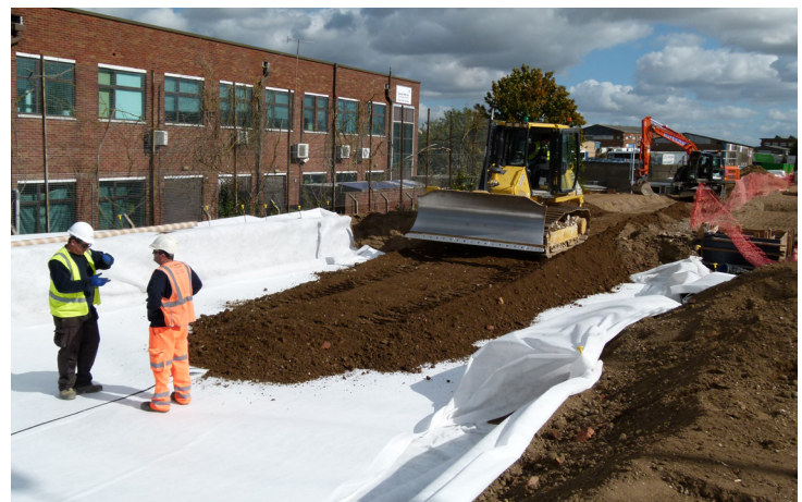
Fildrain covered prior to installation of trunk sections
