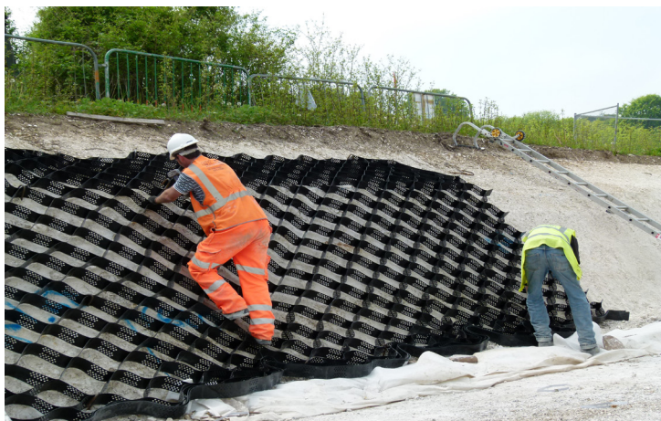
Erosaweb panels installation
