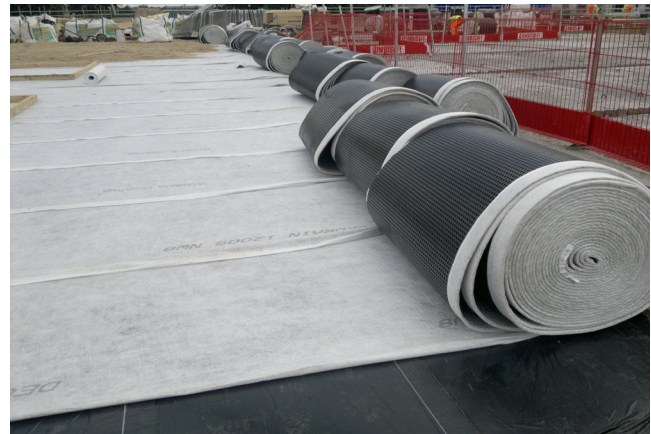
Fig. 2: Rolls of Deckdrain can be quickly laid directly onto waterproofing on concrete roof slabs
