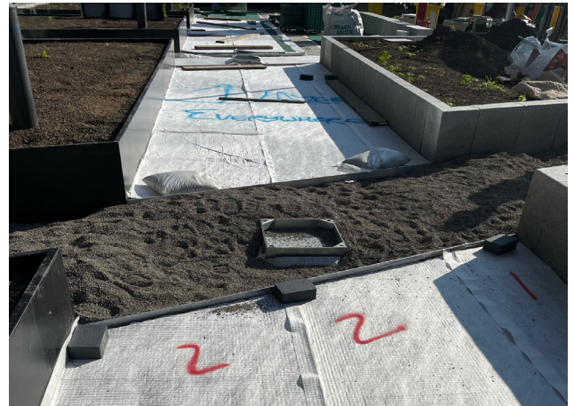
Fig. 12: Non-load bearing walls and planters can be built onto Deckdrain if a suitable concrete footing is cast
