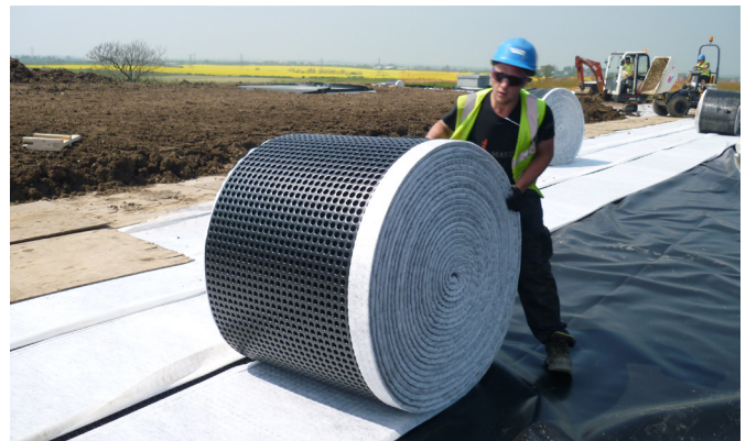
Fig. 5: Install Deckdrain with geotextile facing upwards
