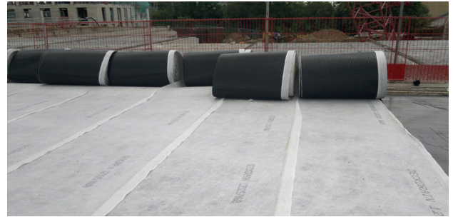
Fig. 8: Deckdrain is butt-jointed and the geotextile overlap prevents soil ingress at the seams
