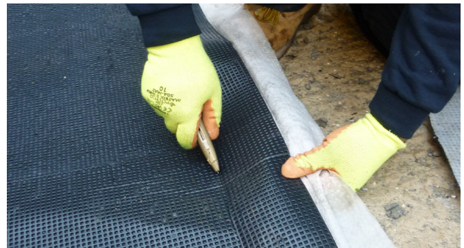
Fig. 6: Cut Deckdrain to length using a safety knife
