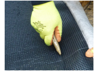
Fig. 1: Roll out and cut Deckdrain with safety knife
