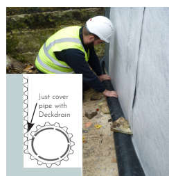
Fig. 5: Position pipe and wrap to just cover the pipe & weight down
