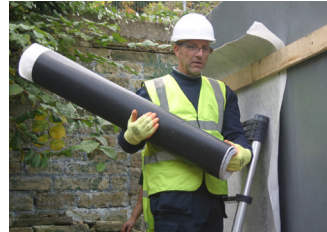
Fig. 1: Roll out and cut Deckdrain with safety knife
