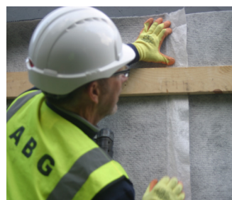
Fig. 2: Hanging the first and second panels. Ensuring overlaps are in place
