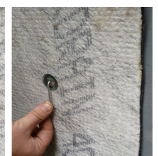
Fig. 4: Alternative fixing method using Abfix stickpins. Remove protective release paper and press the pin firmly to the wall. Surfaces should be clean and dry, free of dust, grease, oil and any other loose matter. Pierce the Deckdrain over the pin, secure in place with the washer and flatten pin.
