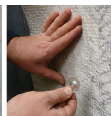
Fig. 4: Alternative fixing method using Abfix stickpins. Remove protective release paper and press the pin firmly to the wall. Surfaces should be clean and dry, free of dust, grease, oil and any other loose matter. Pierce the Deckdrain over the pin, secure in place with the washer and flatten pin.
