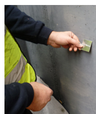
Fig. 4: Alternative fixing method using Abfix stickpins. Remove protective release paper and press the pin firmly to the wall. Surfaces should be clean and dry, free of dust, grease, oil and any other loose matter. Pierce the Deckdrain over the pin, secure in place with the washer and flatten pin.
