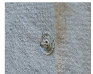
Fig. 3: Fasten midwall with nail and plastic washer
