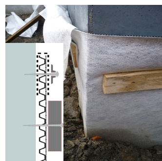
Fig. 11: 300 mm textile tucked behind Deckdrain and overlapped
