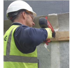
Fig. 2: Hanging the first and second panels. Ensuring overlaps are in place
