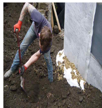
Fig. 10: Shovel soil to level and use a vibrating plate next to the Deckdrain
