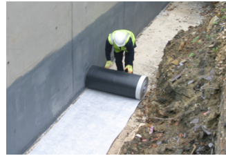
Fig. 1: Roll out and cut Deckdrain with safety knife
