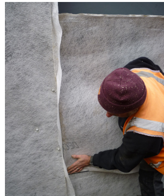
Fig. 8: Place second layer and ensure flaps overlap horizontally and vertically
