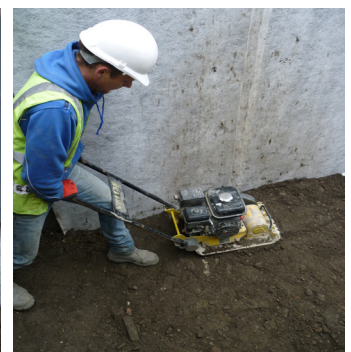
Fig. 10: Shovel soil to level and use a vibrating plate next to the Deckdrain
