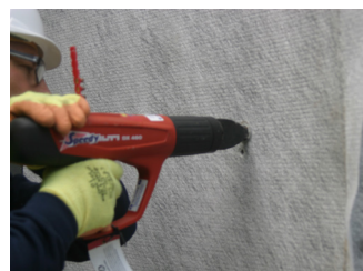
Fig. 3: Fasten midwall with nail and plastic washer
