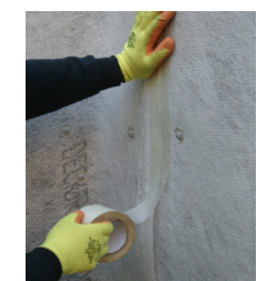
Fig. 6: Seal flaps with ABG jointing tape
