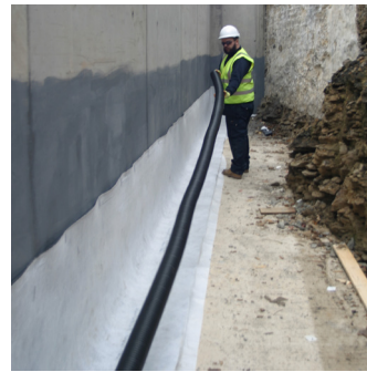
Fig. 7: Roll out Deckdrain horizontally and leave excess material to wrap around the carrier pipe
