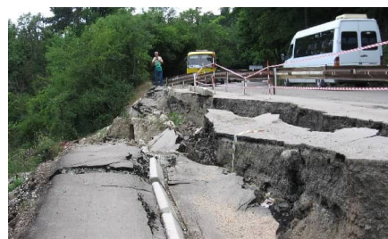
Figure 6: Typical slope failures at roadsides
