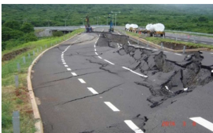
Figure 6: Typical slope failures at roadsides
