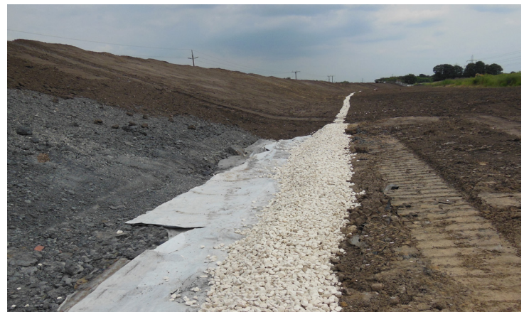
Finished embankment profile with Fildrain tucked into perimeter drain
