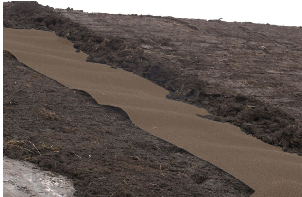
Fig. 12: Place friable topsoil and seed
