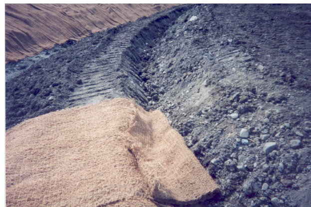
Fig. 9: Place Erosamat at the base of the anchor trench
