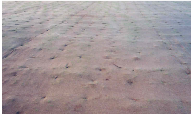
Fig. 10: Pin into place at 1m centres or as specified on the drawings. Insert additional pins into any hollows / undulating ground
