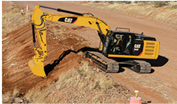
Fig. 7: Smooth out slopes using a grading bucket or blade
