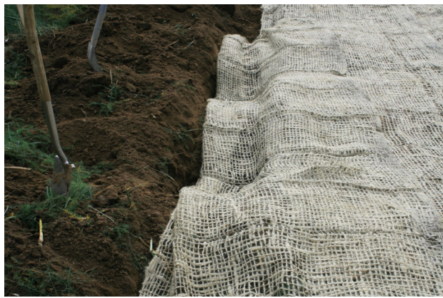
Fig. 11: Pin to toe and side trenches where required
