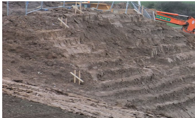
Fig. 8: Steeper slopes may require shallow benching
