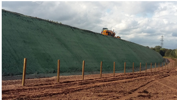
Fig. 13: Hydroseeding of steep slopes
