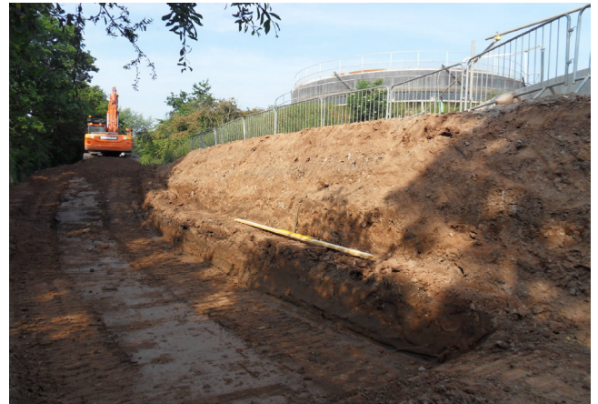
Fig. 1: Prepare slope to create an even surface
