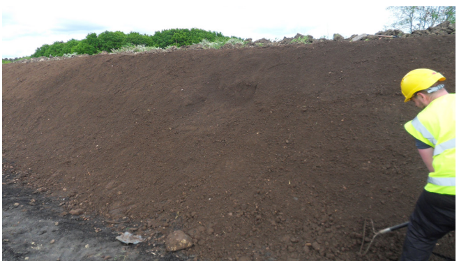
Fig. 6: Rake in 10mm cover of friable topsoil
