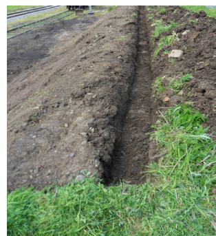
Fig. 2: Excavate anchor trenches
