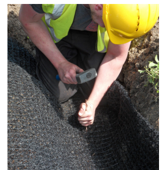
Fig. 3: Pin Erosamat into anchor trench
