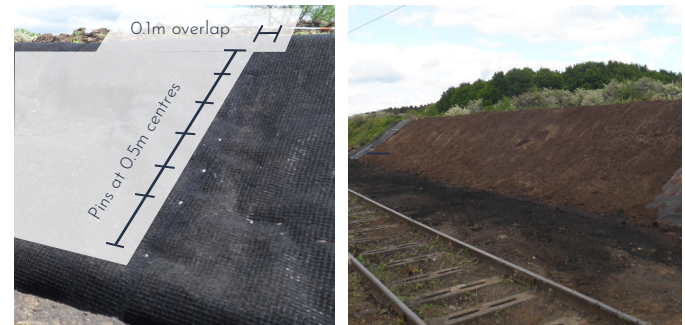
Fig. 9: Cross-slope overlaps and pinning
