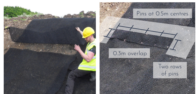
Fig. 8: Downslope overlaps and pinning
