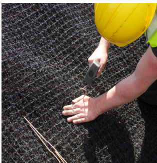
Fig. 4: Pin Erosamat to slope
