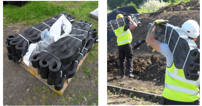
Fig. 1: Delivery of and carrying panels
