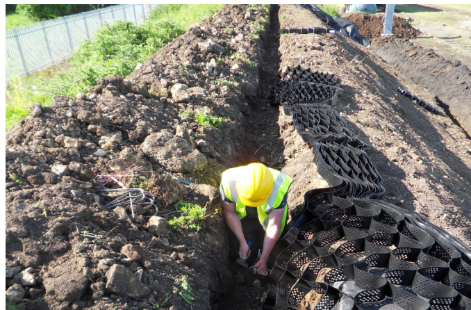
Fig. 4: Place Erosaweb and pin into anchor trench
