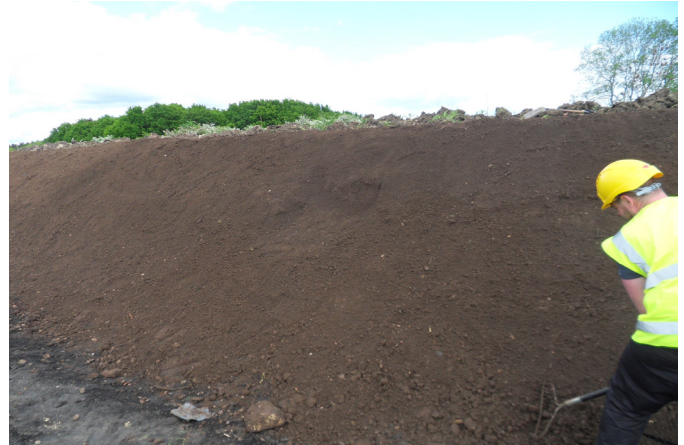
Fig. 8: Place topsoil from bottom up
