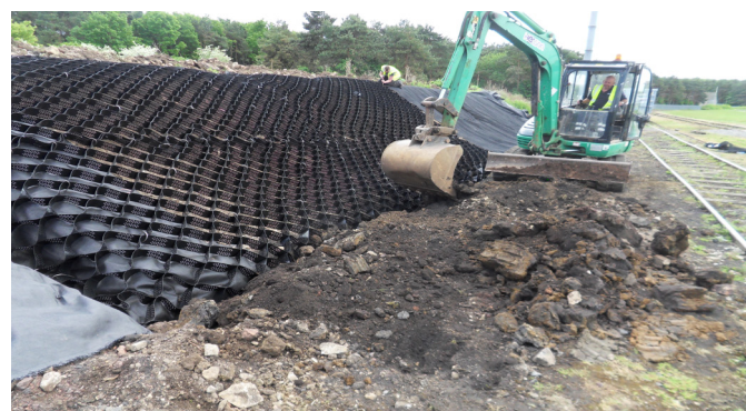
Fig. 7: Backfill all trenches
