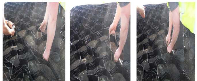
A) Remove pin at base of panel
