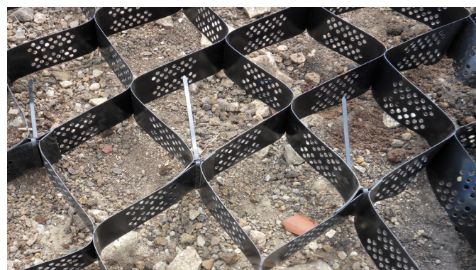
Fig. 6: Connect Erosaweb panels with cable ties
