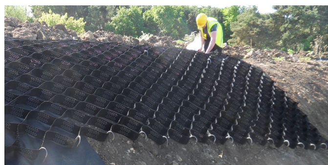
Fig. 5: Expand Erosaweb down-slope and pin in place
