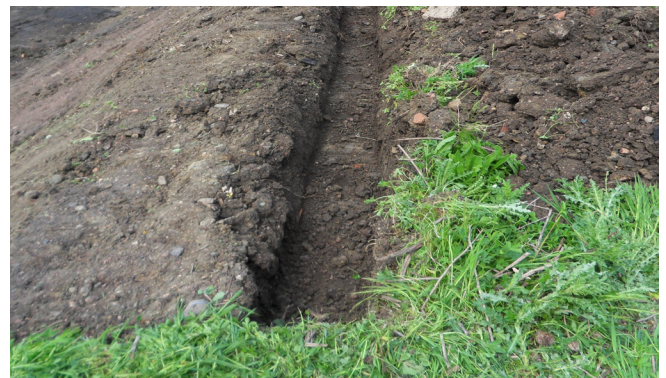
Fig. 2: Excavate anchor trenches
