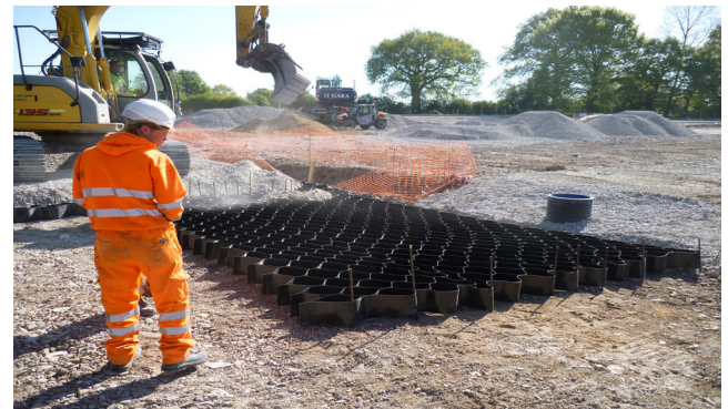
Fig. 6: Erosaweb TRP fully pinned into position
