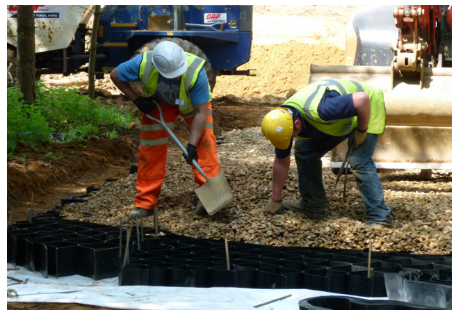
Fig. 7: Webs being backfilled
