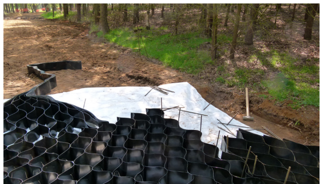
Fig. 4: Erosaweb TRP being stretched into position
