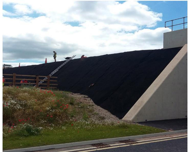
Erosamat 3/20Z500 installed on railway embankment
