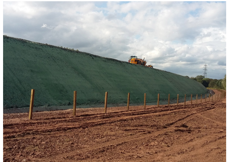
Hydroseeded Erosamat erosion control system
