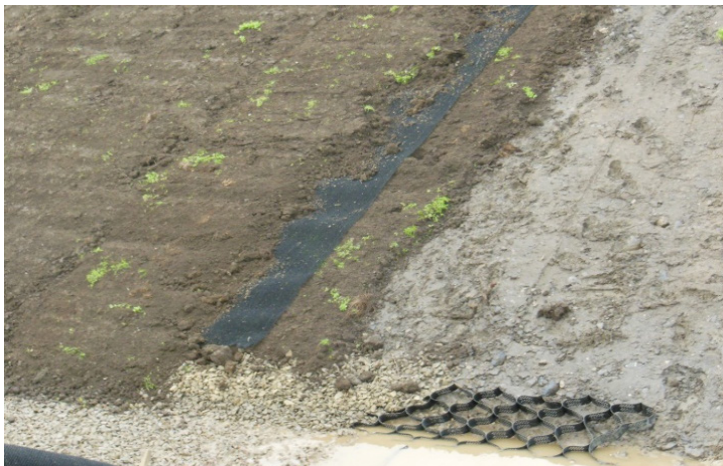
Erosamat (slope) & Erosaweb (base) used in combination to form a complete geosynthetic solution
