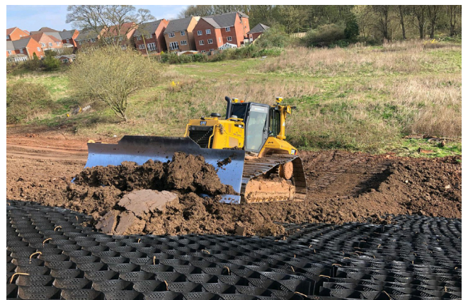
Backfilling Erosaweb panels using bladed dozer
