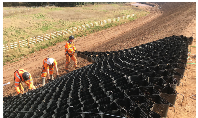
Expanding ABG Erosaweb panels into position & pinning
