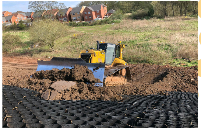
Backfilling Erosaweb panels using bladed dozer
