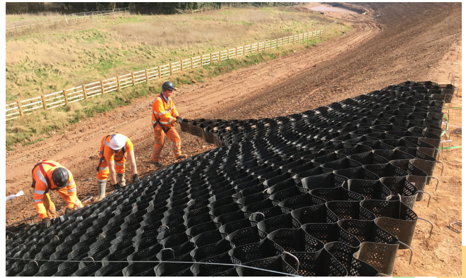
Expanding ABG Erosaweb panels into position & pinning
