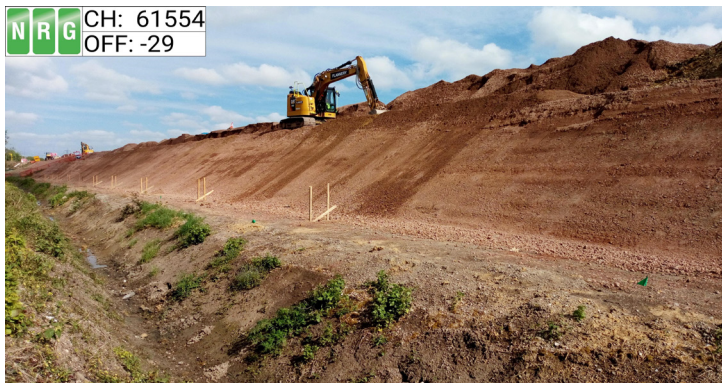
Widening and re profiling of the embankment at M4 J12
