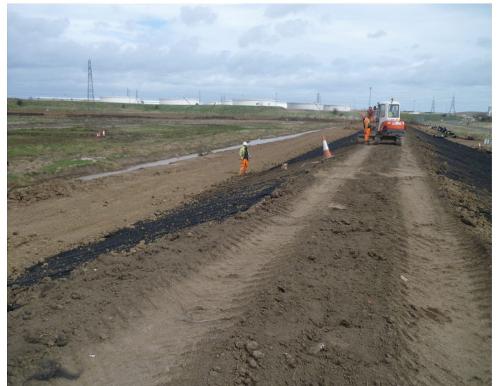
Topsoil filling of Erosamat
