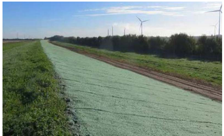
The highest risk areas were hydro seeded to accelerate vegetation establishment
