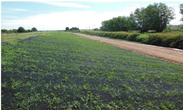
Natural vegetation binding with Erosamat and blending with the natural environment
