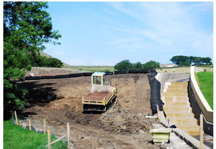
Steep slope with 6m/s design flow rates
