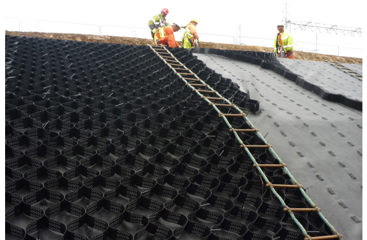
Erosaweb placed in anchor trench and expanded down slope
