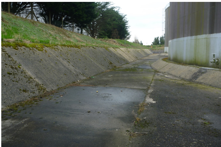
Existing bunds to be lined and extended
