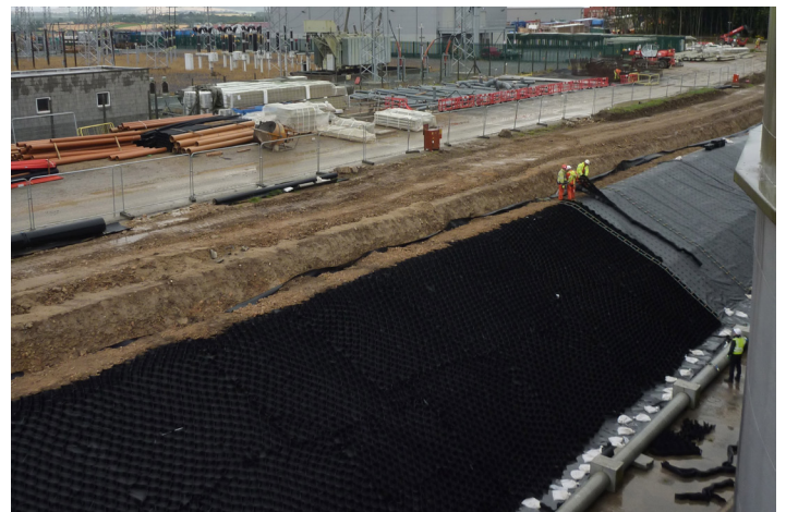
Erosaweb anchored in place ready to receive topsoil
