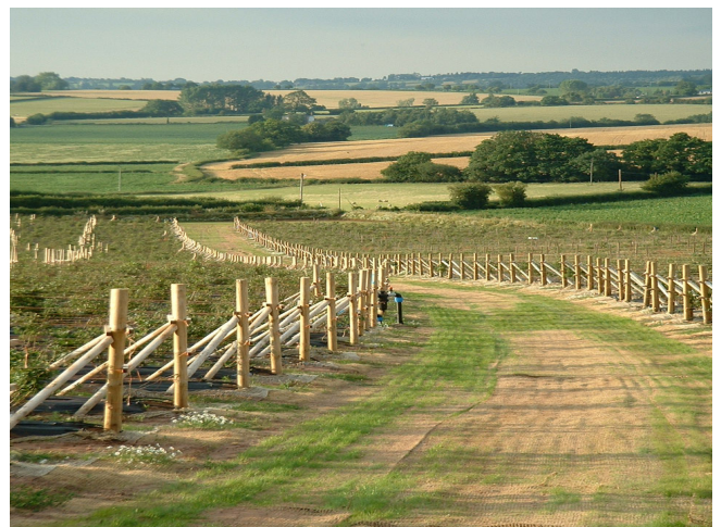
Partially established grassed waterway
