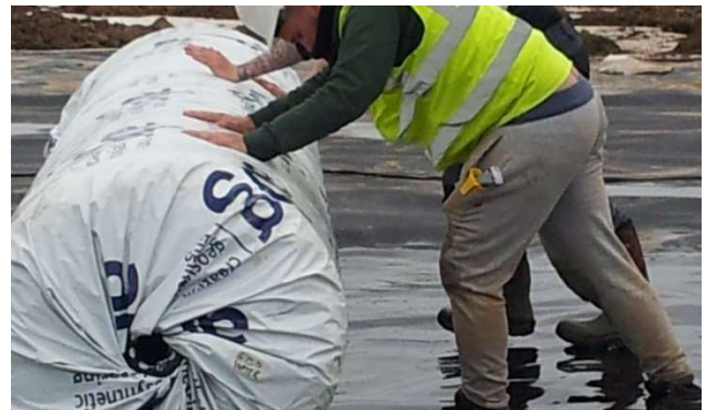
Fig. 3: Moving rolls around site
