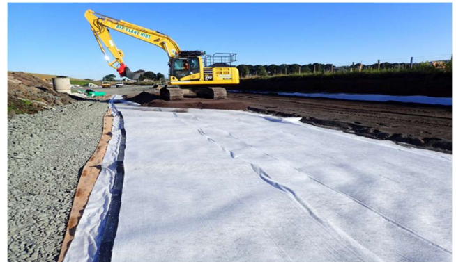
Fig. 8: Site plant operating on layer of backfill
