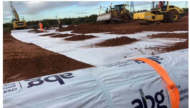
Fig. 1: Fildrain partially backfilled
