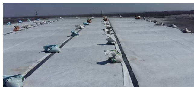
Fig. 6: Using sandbags to prevent wind uplift
