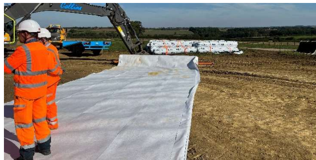
Fig. 5: Unrolling Fildrain onto firm formation
