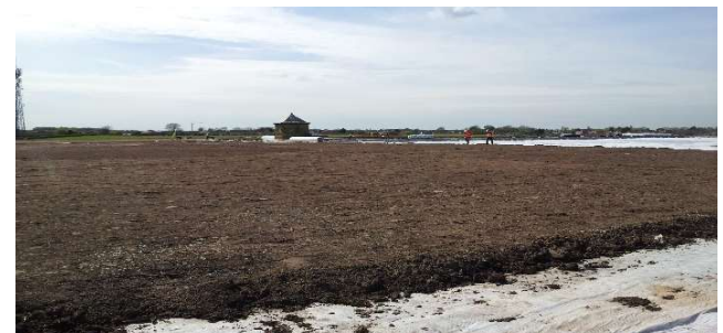
Fig. 9: First layer of backfill laid
