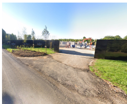
Site entrance prepared and ready for surfacing.
