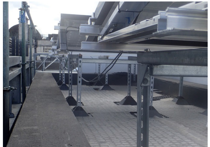
The versatile ABG Roofdrain geocomposite was fitted around footings of the PV arrays to form a continuous drainage layer
