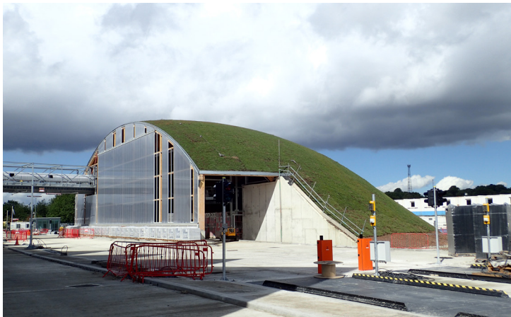
Finished lightweight ABG Green Roof System
