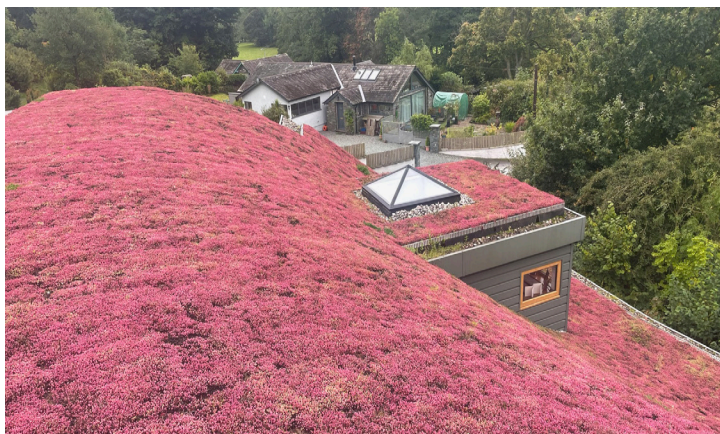
The sedum extensive green roof in Autumn
