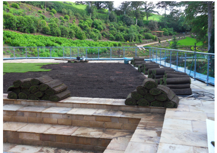
Final installation of turf onto the terrace
