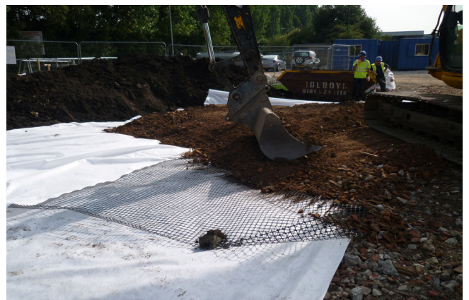
Terrex geotextile and Abgrid geogrid supporting 6F2 hardcore over soft ground
