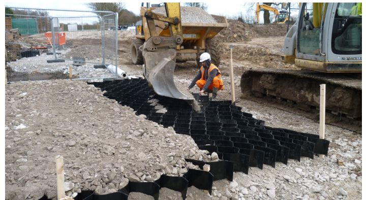
Abweb can provide a 50% reduction in the required thickness of sub-base
