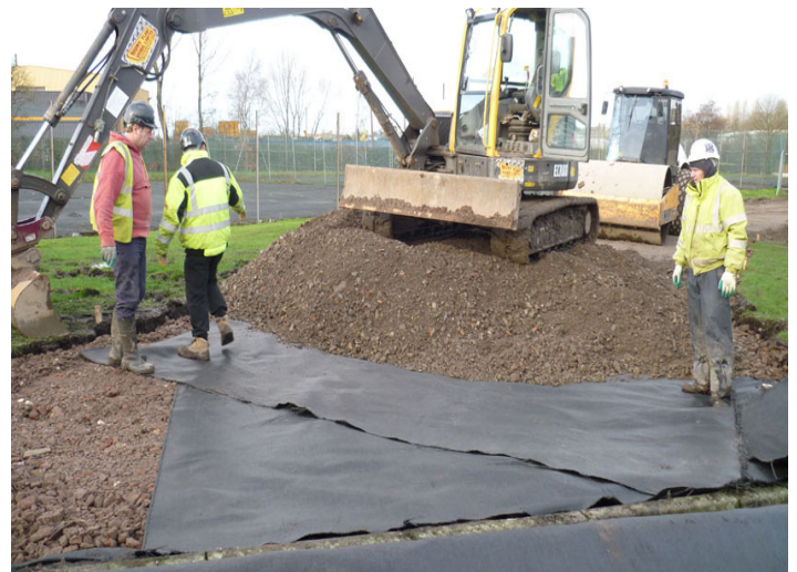
Installation of Gridtex reinforcement layers
