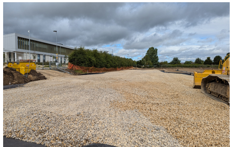
Stabilised and separated layer of SHW Series 800 Type 3 sub-base
