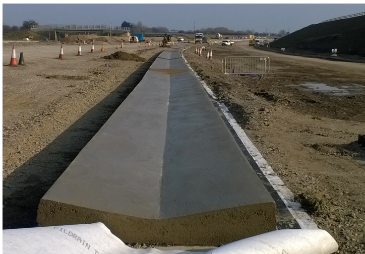
Channel extruded directly onto ABG Fildrain Type 10
