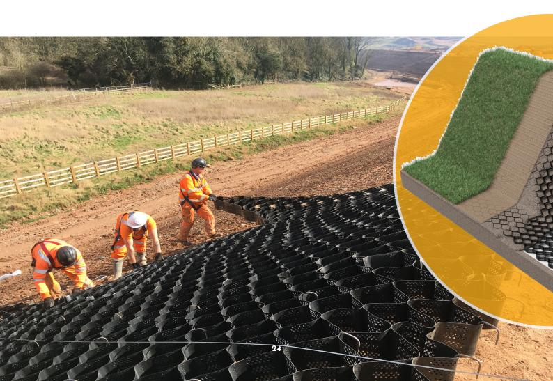
**Erosaweb®** geocell is designed for the reinforcement of weak soils and has many applications, including the retention of soil onto steep profiled sections of highway embankments. The cells of the geocell retain the fill material whilst still permitting water to drain through.
