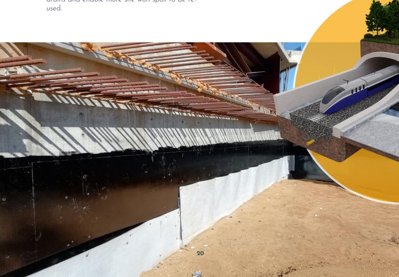
**ABG Roofdrain®** geocomposite layers can be utilised for green bridge applications to provide a combined water reservoir and structural drainage function, supporting vegetation growth and protecting the bridge deck waterproofing respectively. Available with different core thicknesses and geotextile options to suit the specific loading conditions.
