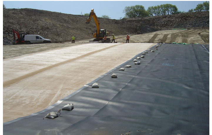
Double lining system installation GCL and 2mm textured HDPE geomembranes
