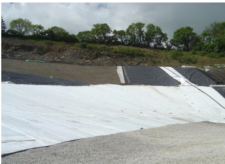
Pozidrain Protector puncture resistance to deliver geomembrane protection at 45m depth
