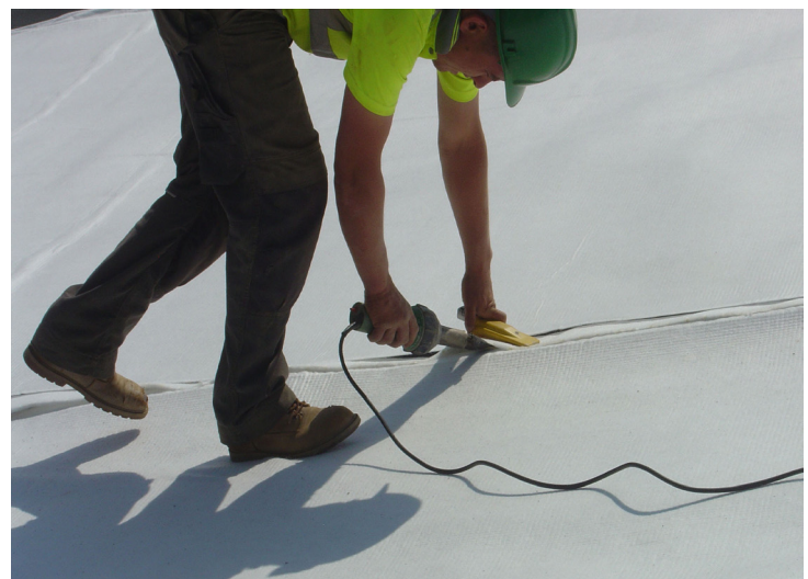
UV resistant Pozidrain geotextile tack welding with a hot air gun
