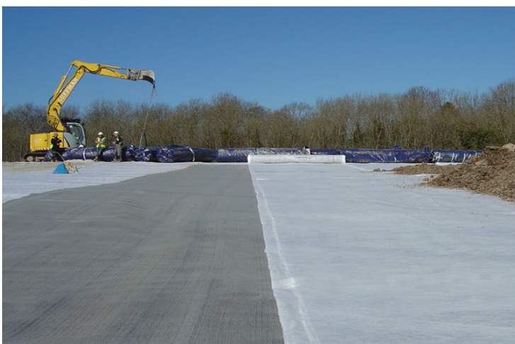
Claymat GCL installed between Pozidrain geocomposites
