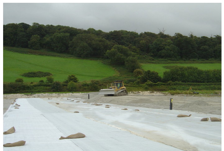
Adequate interface friction ensured slope stability
