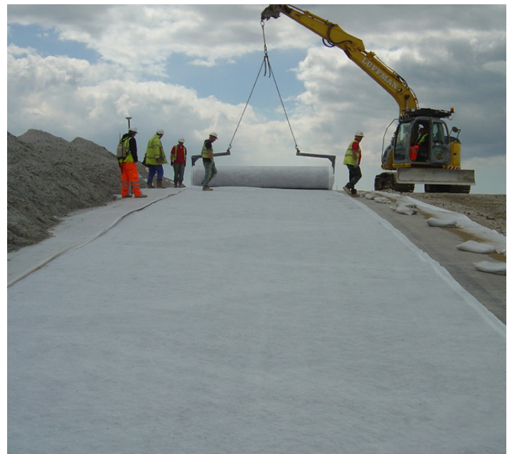
Large Pozidrain rolls enabled rapid installation
