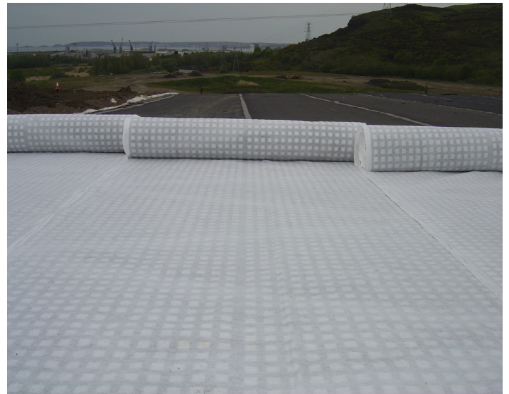
Wide-width rolls enabled rapid installation
