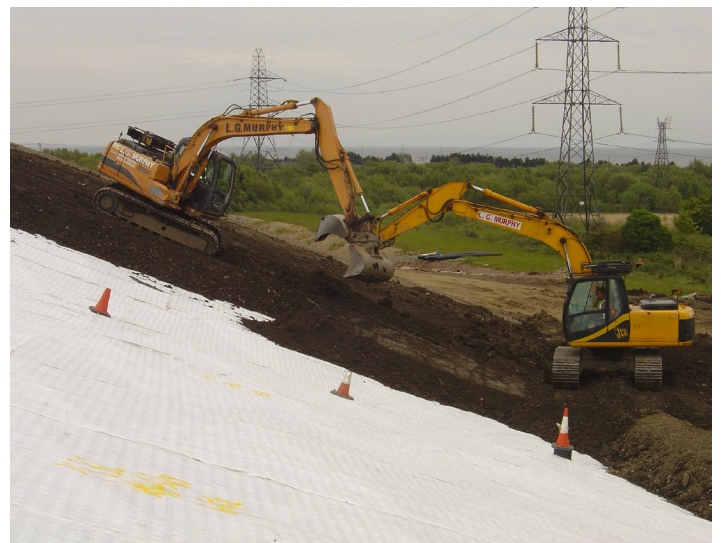
Superior interface friction ensured 1 in 3 slope stability
