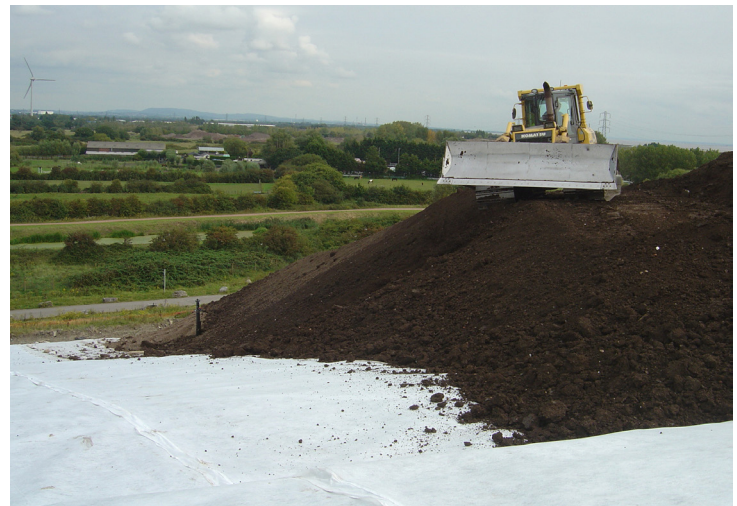
Superior interface friction ensured slope stability
