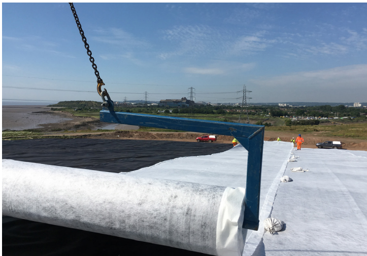
Pozidrain installed on top of 1mm LLDPE textured liner
