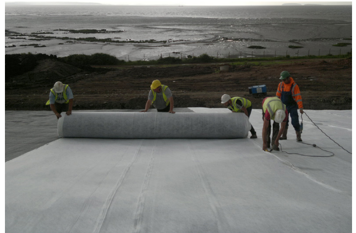
Wide-width rolls enabled rapid installation
